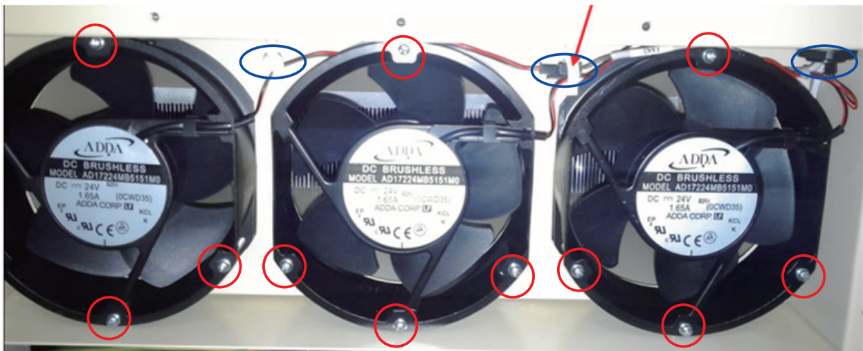
Figure 80. Remove Power wires and Fans
